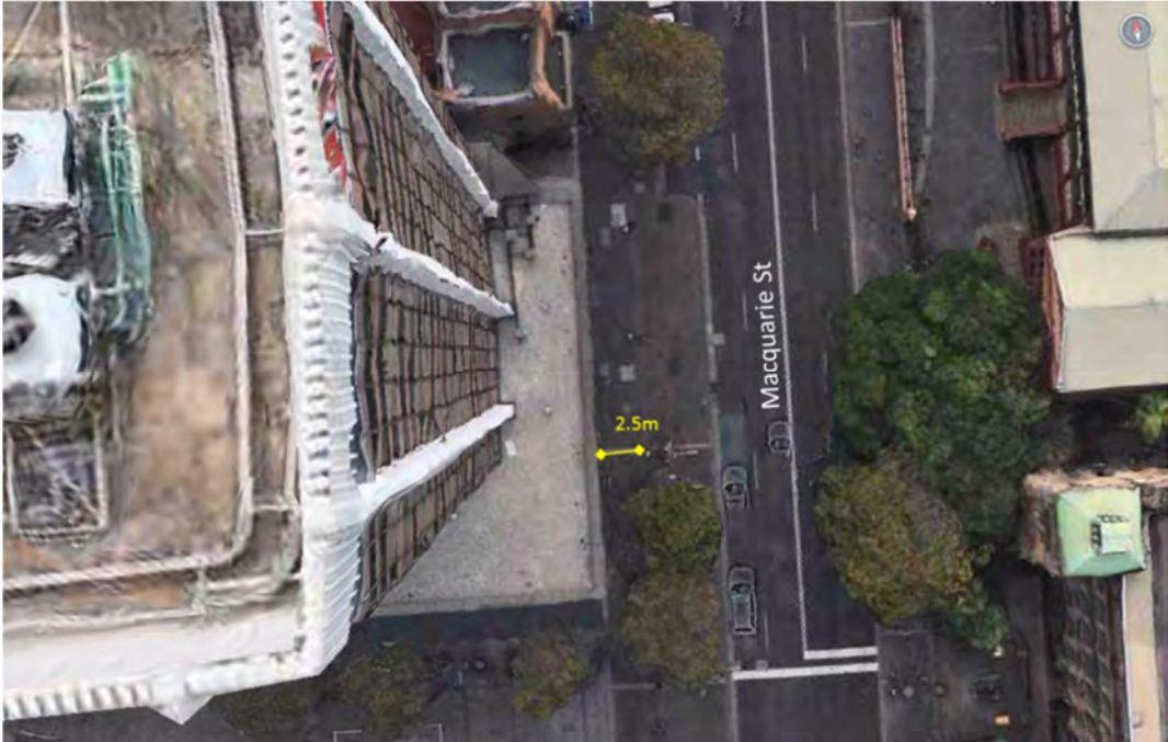
Figure 11 - Clear footpath width in Macquarie St frontage
